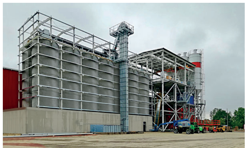
General view of batching plant under construction
