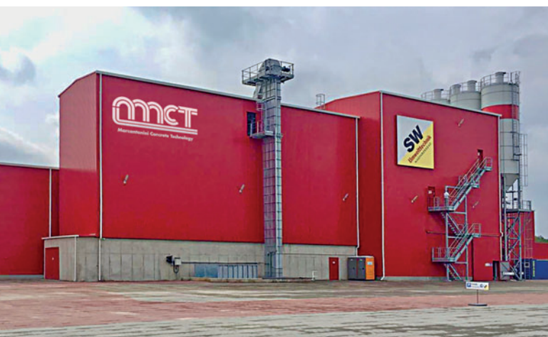
General view of batching plant after completion
